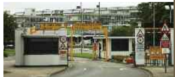
Boots PLC aka Holyhead ferry terminal
